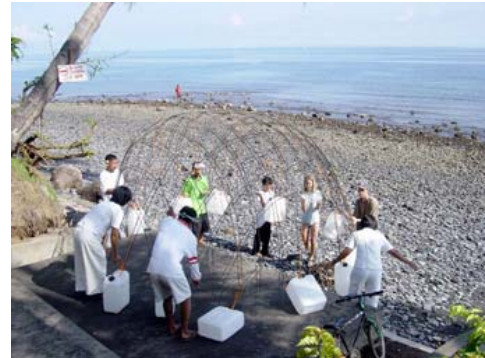
Figure 7. BioRock™ “dome” structure after assembly in Bali, Indonesia (Ref. Dr. Thomas Goreau)
