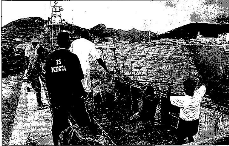
About four Scouts helped to build the framework for a manmade reef using Biorock technology at Bobby's Marina on Thursday. This John Halley photo shows the frame being placed into a boat to be transported to another location where it will be placed underwater.
