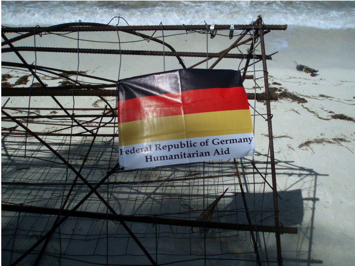
Figure 3. A Biorock shore protection module, made from welded steel bars with shelves for growing corals and giant clams, waiting on the beach to be installed.
