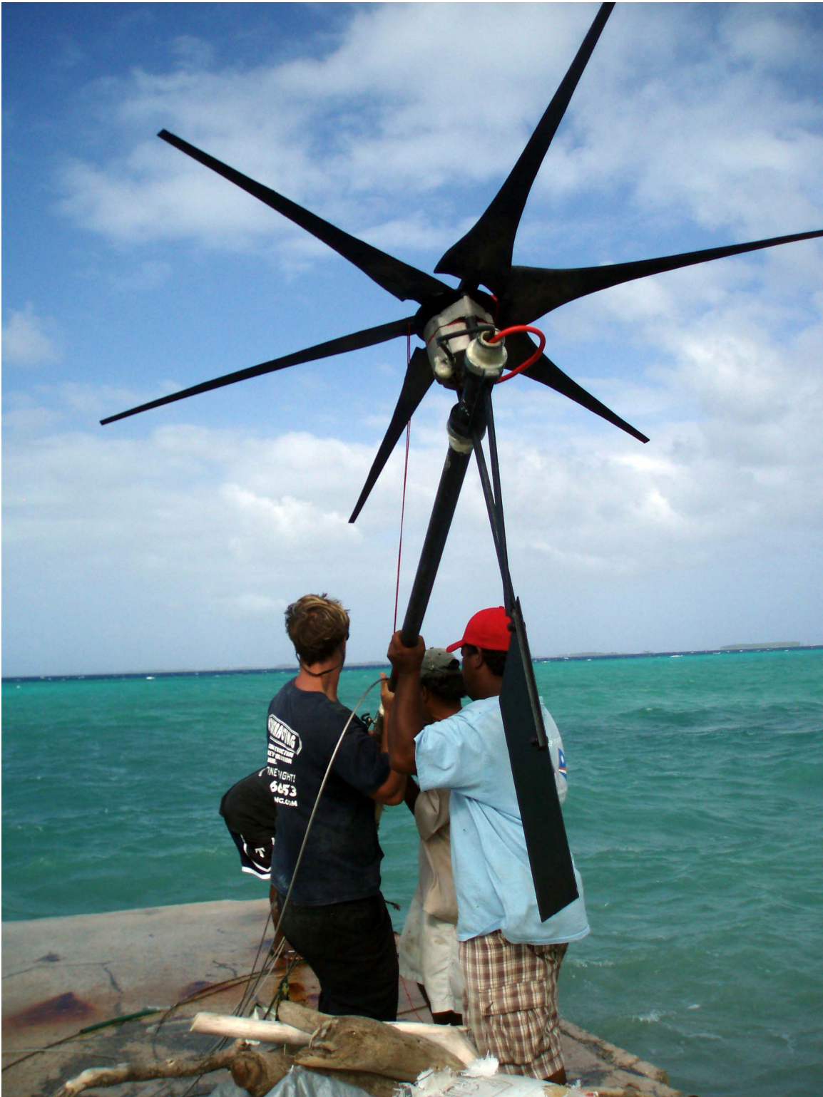
Figure 4. Installing the replacement windmill.
