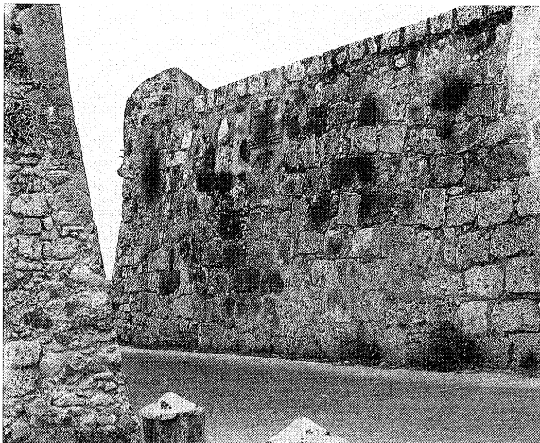
View of a coral-stone wall built more than three hundred years ago in Cartagena, Colombia. The coral stones were formed with the same chemicals as the ones suggested for the seawater concrete.
