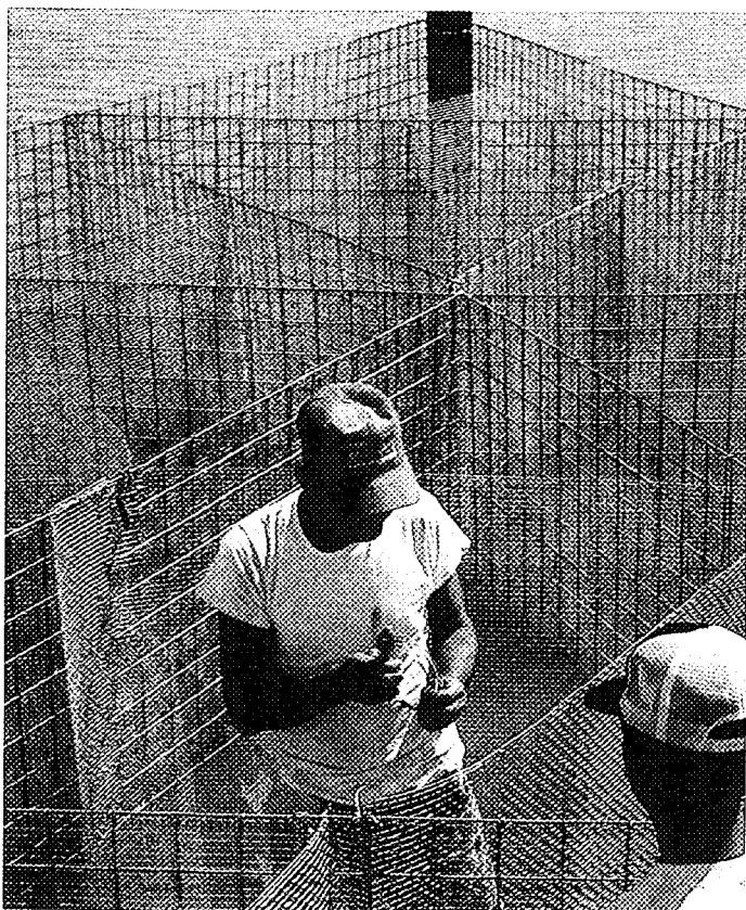
Another important use of mineral accretion is in forming artificial reefs as a tool for increasing fish populations. Wire mesh of different gauges is particularly well-suited to this end. This is a view of a demonstration artificial reef constructed by Hilbertz in St. Croix in 1976.
