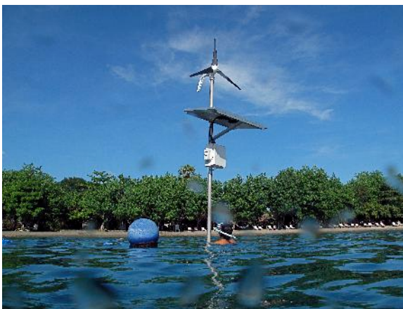
Biorock structures powered by wind and sun (left, Bali, by Rani Morrow-Wuigk), or by wave generators (right, Marshall Islands, by Tom Goreau).
