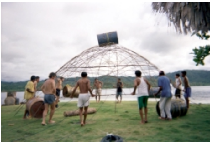
Lifting the dome-shaped Akuabiski Galu coral nursery on Iskardup
