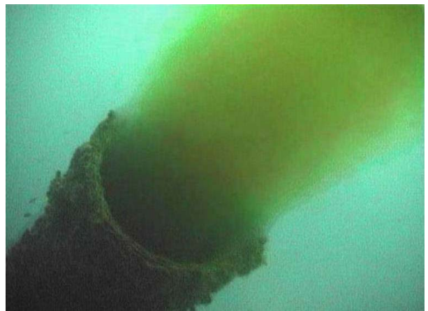
SLOW DEATH: A pipe 90 feet underwater and about a mile offshore discharges 13 million gallons of partially treated sewage each day.
