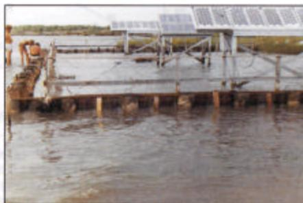
4. A growing spoil containment structure in the Gulf of Mexico. Photovoltaic panels were used as a backup to drive mineral accretion during frequent power outages. Photo: W.H. Hilbertz.
