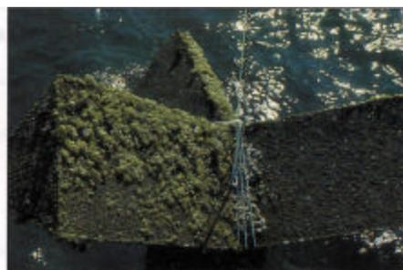
2. Cathodic building component shown in Photo 1 during accretion phase. Photo: W.H. Hilbertz.
