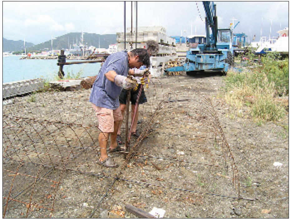
Building the structure.
