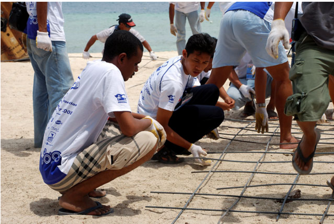
3. Tying steel bars together to form structures
