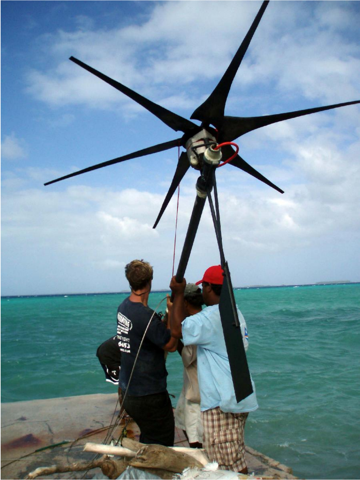
Figure 4. Installing the replacement windmill.
