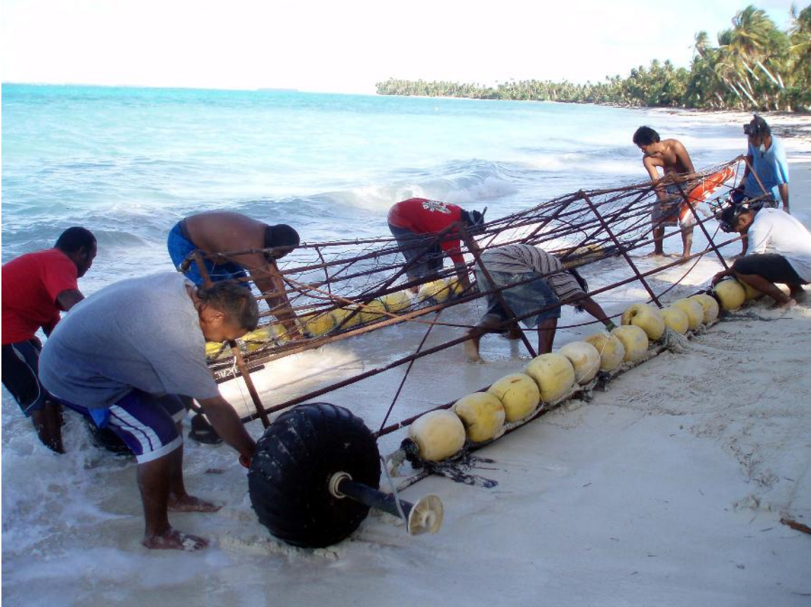
Figure 13. Preparing floats to move module to the correct location.
