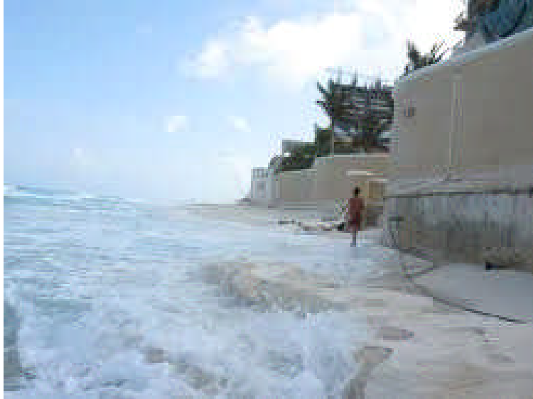
Figure 5. Cancun seawalls cause beach erosion, causing endless cycles of sand dumping, all of which washes away again (Google images)
