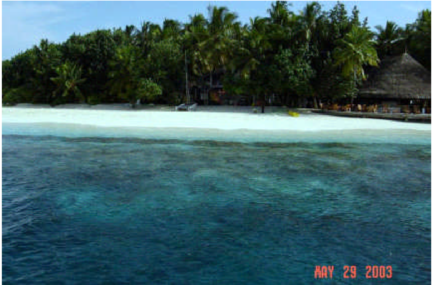
Figure 11. New Beach grown in two years at Ihuru Island, North Male Atoll, the Maldives, at a location where the beach had eroded away and the building on the right was about to collapse into the sea at the start of the project. The Biorock shore protection reef is the dark line in front of the beach. The Asian Tsunami passed right over this island without causing any damage to beach or reef. Photo by Azeez Hakeem.
