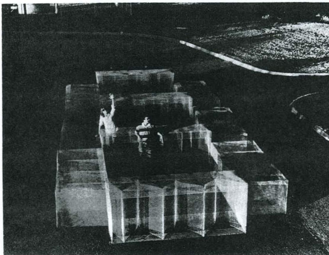
Fig. 17. Artificial Reef 4 assembled on land.
