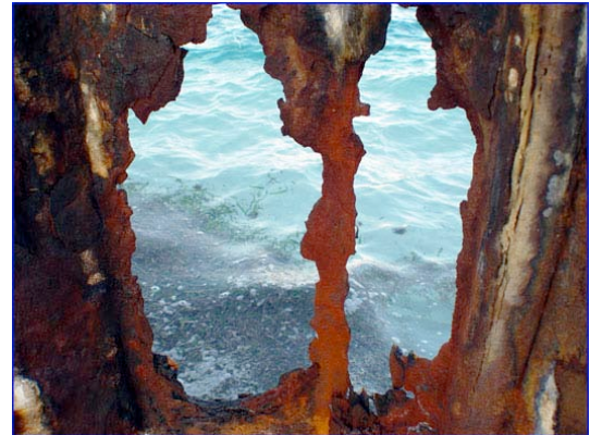
Rusting sheet metal piling
