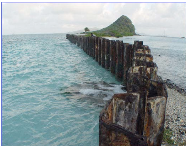
Sheet metal piling and causeway restricting the flow of water into the lagoon near Frigate Island
