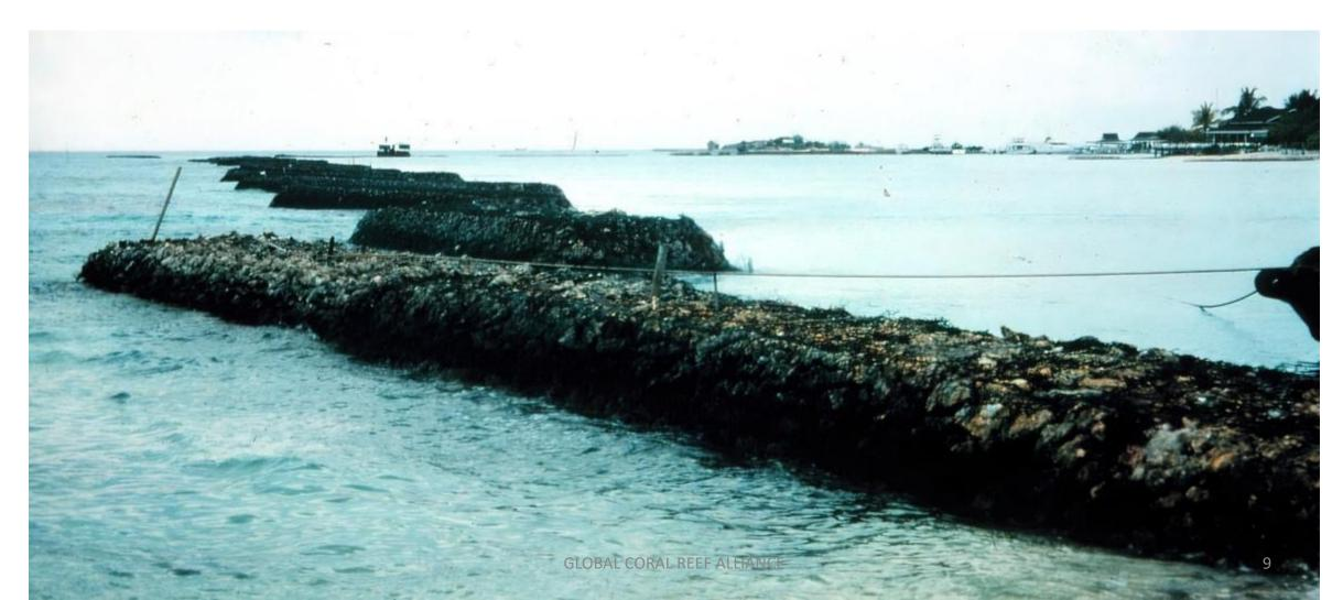
These seawalls reflect waves and cause sand to be scoured away in front of, and then underneath them, until they eventually collapse. Photograph 1996 by Wolf Hilbertz.
