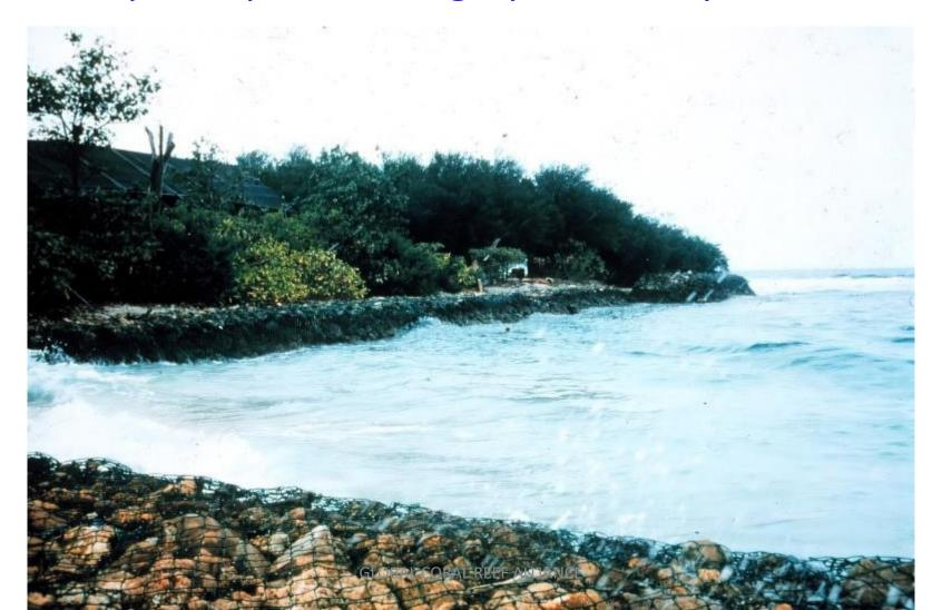
Expensive plastic coated wire soon cracks in ultraviolet light, and the rusting steel stains the limestone. Photograph 1996 by Wolf Hilbertz
