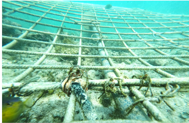
Raccordement : câble/cathode
